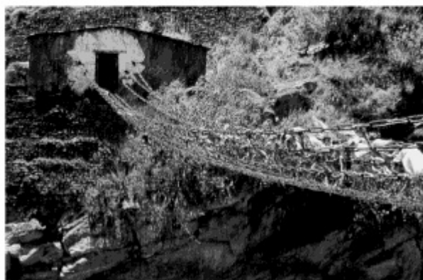
Fig. 20. Iron chain suspension bridge at Duksum, Tashigang ( bla shis gang ), eastern Bhutan, built by Tangtong Gyalpo, early 15th century. The walkway was probably formed from wooden slats, which no longer exist. Lines of multiple chains forming the sides and path supports are secured within the massive stone gatehouses at either end (photo: the author, 1998)
